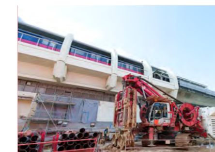
Pasir Ris 8 Singapore Low headroom diaphragm wall with HC05
