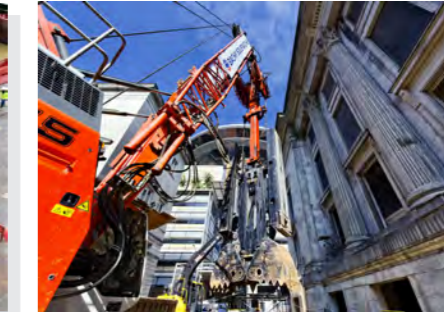
National Gallery Singapore Construction of diaphragm wall in confined space
